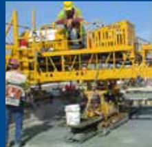
I-95 Deck Rehabilitation
