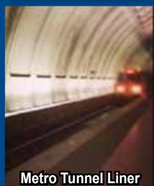
Metro Tunnel Liner
